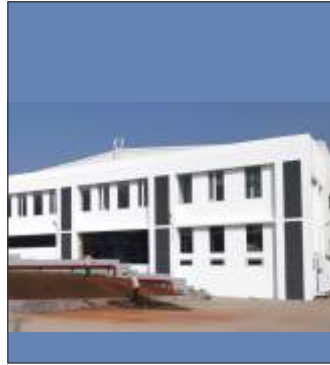
PHOENIX MECANO (I) PVT. LTD. Area - 60,000 Sq. Ft. Cost - 600 Lacs Architect - Archicon Associates, Pune Location - Urse, Tal. Maval, Pune
