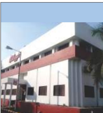
KELLOGGS INDIA LTD. Area - 6000 Sq. Ft. Cost - 275 Lacs Architect - Designer Sanyojika Location - Talaja Mumbai
