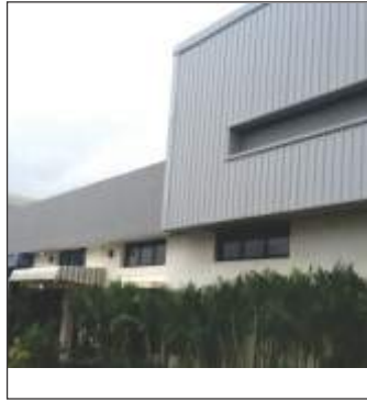
PHOENIX MECANO INDIA P. LTD. Cost - 200 Lacs Location - Pirangut, Pune
