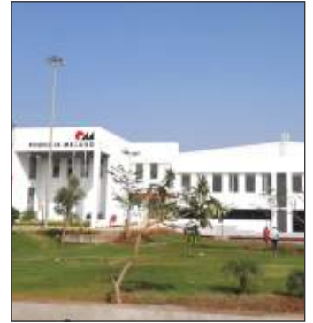
PHOENIX MECANO INDIA P. LTD. Area - 1,00,000 Sq. Ft. Cost - 1200 Lacs Architect - Archicon Associates Location - Urse, Pune
