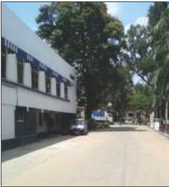
EXIDE INDUSTRIES LTD. Positive Expander Unit Expansion of Factory Building & Road Cost - 1.50 Cr
