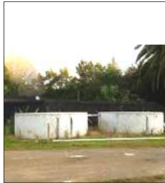
EXIDE INDUSTRIES LTD. UGWT & Road Cost - 107 Lacs Consultant - P K Associates Location - Talaja
