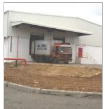
AVERY DENNISON INDIA PVT. LTD. Industrial Project Area - 20,000 sq.ft | Cost - 200 lacs Consultant - C.R.Narayan Rao, Chennai Location - Ranjangaon MIDC, Nagar Road, Pune.
